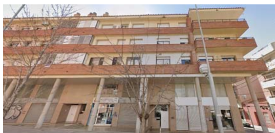
Residential (Terrassa, Spain)
